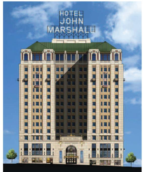
Today, extensive construction got under way on the existing historic building to renovate and transform it to a modern, functioning historic landmark. The exterior construction renovation will begin with replacing all windows with more energy-efficient ones, restoring the ornamental work and gold gilded accents, replacing the sloped standing-seam roof, and restoring the rooftop lit name back to its original luster.
