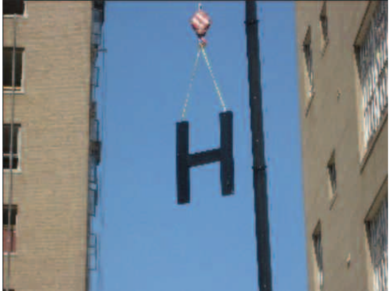
An "H" starts its journey to the top of the Hotel John Marshall building in an alley between Grace and Franklin streets.
