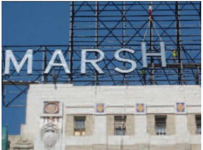
Workers secured an H on the old Hotel John Marshall sign today after it was lifted to the top of the 16-story building by crane.
